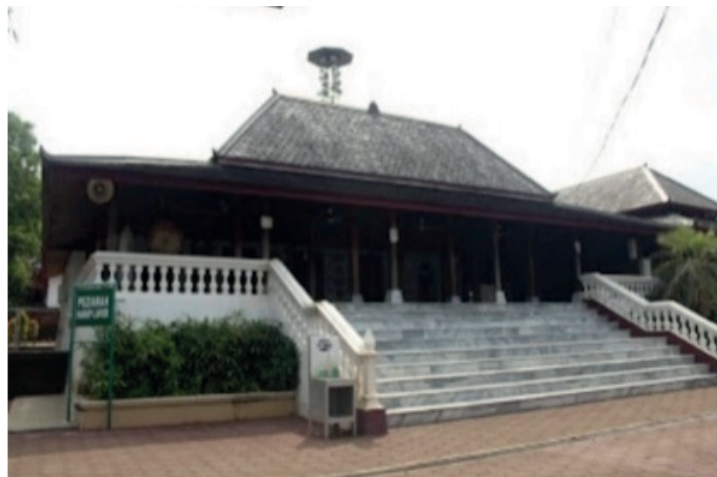
Figure 1: The Masjid Mantingan.
